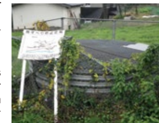
Collecting wells (Wells for draining)
